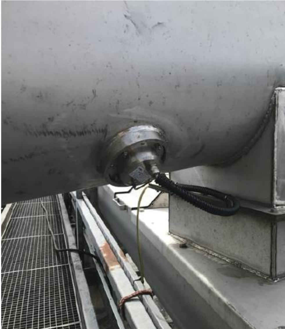
A sensor mounted at the bottom of the main screw conveyor
