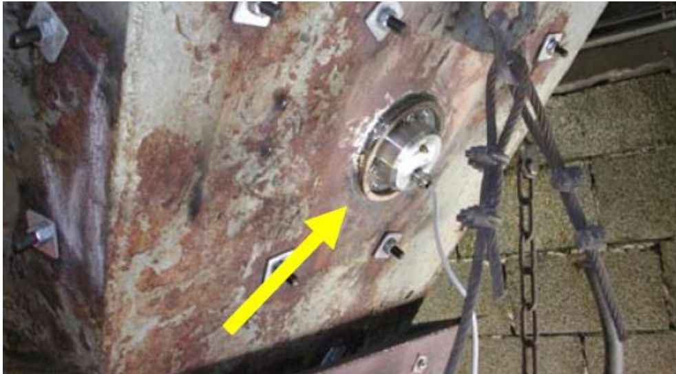
A Humy measures the moisture of coke in a chute
