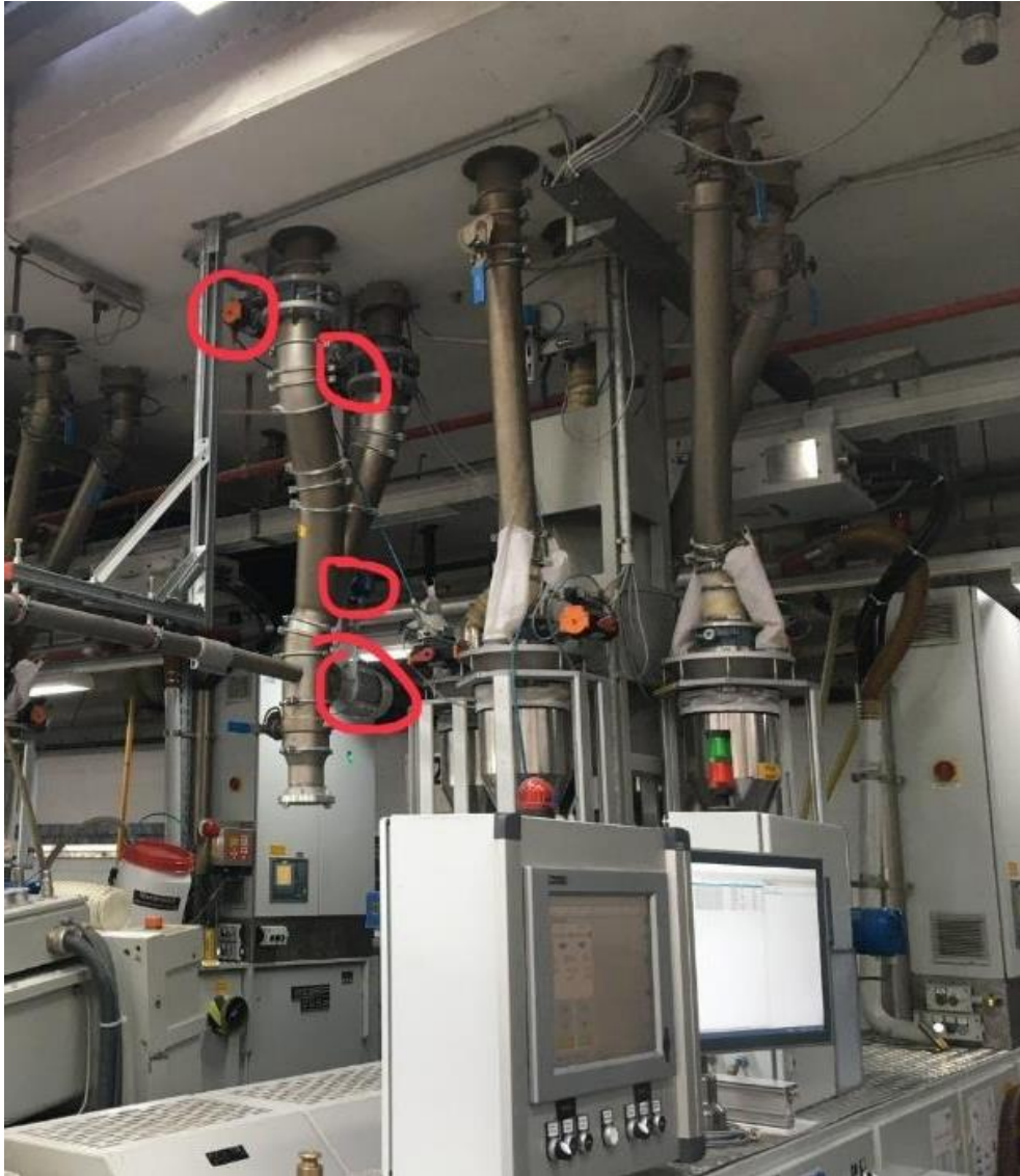
Humys are installed in the pneumatic pipelines
